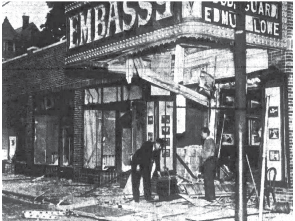
Bombed out theater: Patrolmen Edward Coffey and Herb Olsen search through the debris outside the theater (Photo: The Herald Statesman)
