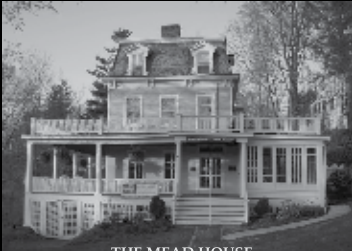
THE MEAD HOUSE 12 ELM STREET DOBBS FERRY, NY 10522
