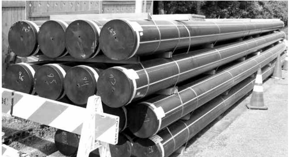
A stack of 12-inch reinforced HDPE gas main pipes awaiting installation and burial to replace old iron pipes in street sections of Con Edison's network on the eastern side of Dobbs Ferry. The mains connect to smaller HDPE pipe inside homes and businesses. State regulations mandate the replacement schedule. Pipe shown is forecast to last more than three times as long as metal pipe.
