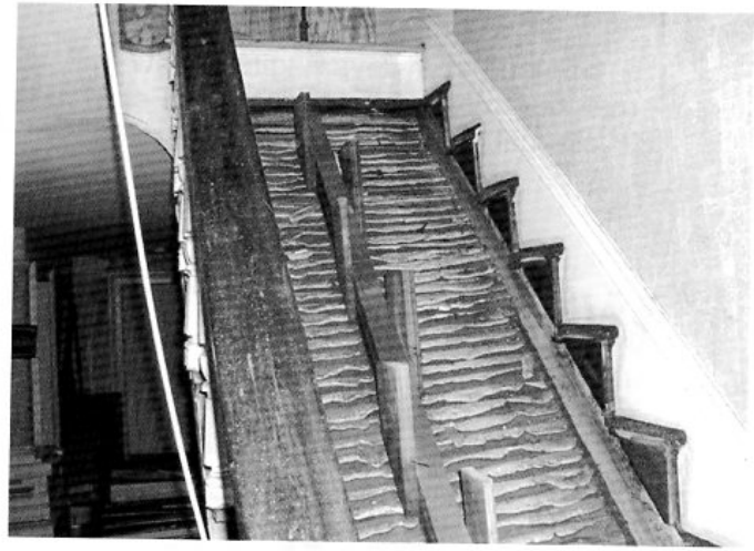
Mead house stairwell repair in progress
