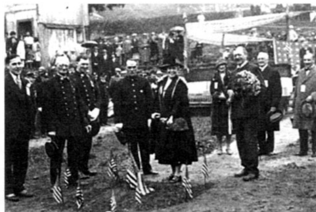
Surrounded by officials from the village, firefighters and police, Mrs. Franklin Q. Brown breaks ground for the new Village Hall
