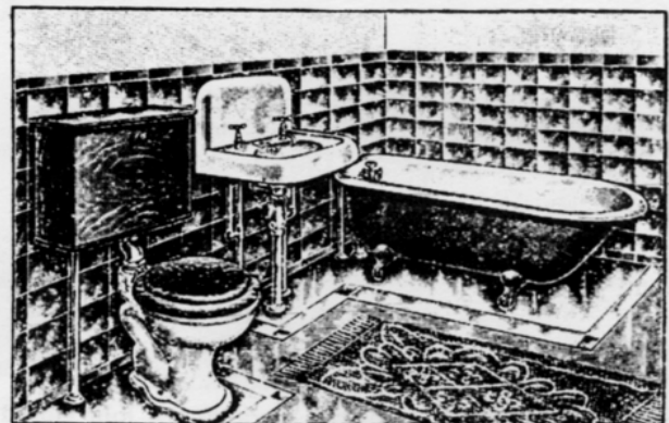
Brand new inside plumbing in 1883 frequently made problems outside.
